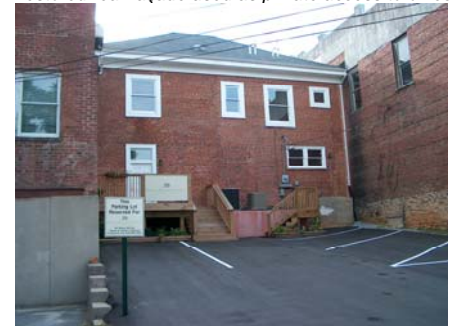
Restored rear facade used as private access to offices.
