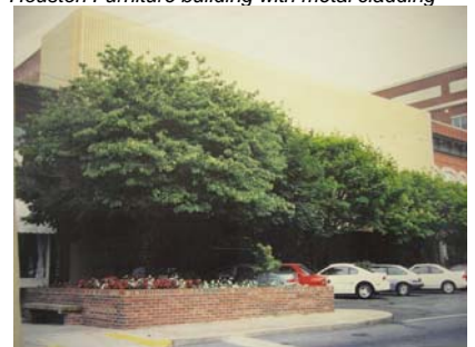
Houston Furniture building with metal cladding
