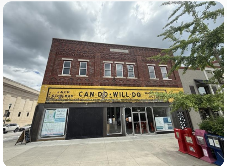
344 N Main Street's facade rehabilitation was approved by the Historic Preservation Commission this year.
