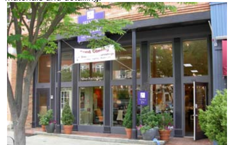
This new storefront uses traditional wood materials and detailing.
