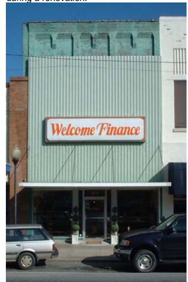
The brick corbelling of the historic façade is still visible above the metal skin applied during a renovation.
