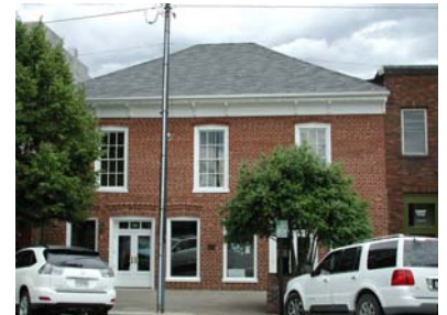
Retain and preserve original windows and doors.
