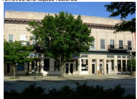
Houston Furniture building after metal cladding removed and façade restored
