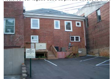
Restored rear façade used as private access to offices.
