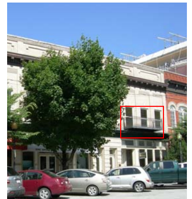
Restored balcony reflects the size and material of historic balcony.
