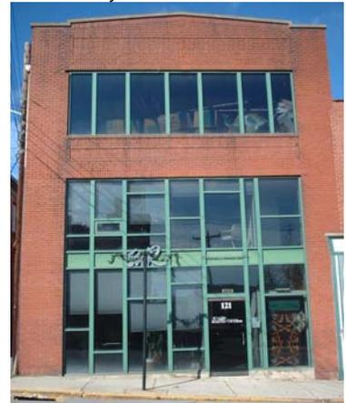
*The utility meters should have been located on the side wall rather than the street façade.*
